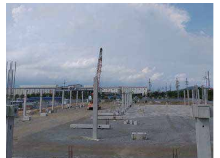
Precast Beam & Column Installation
